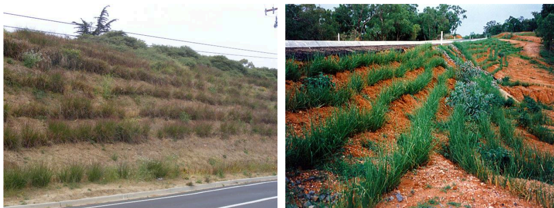
Figure 12. Vetiver is used to stabilize roadsides in California (left) and Australia (right).
